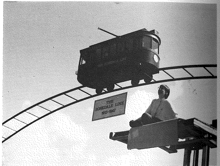
RDA Executive Director inspects the Rosedale Line at Hennessey Sheet Metal
