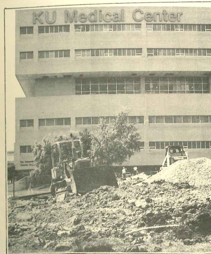
Construction begins on KUMC's new biomedical research building.
