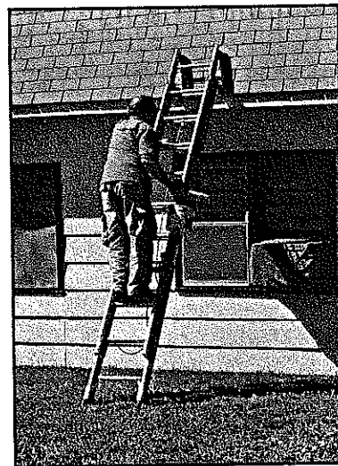
A volunteer prepares to paint a house in Rosedale.
