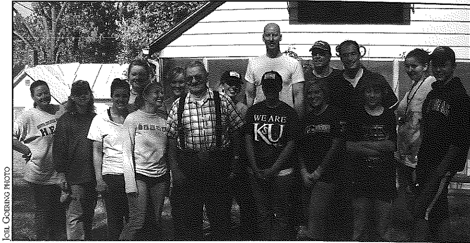
This friendly group of volunteers made repairs at the home of Marvin Orndorf (man with suspenders in middle) during Rosedale's Christmas in October project.
