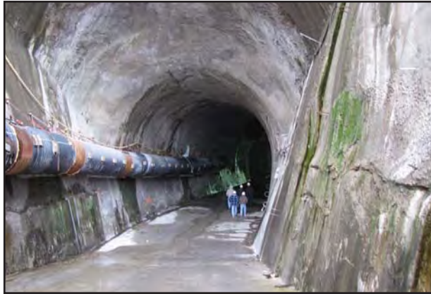
U.S. Army Corps of Engineers Turkey Creek Flood Control Diversion Tunnel
