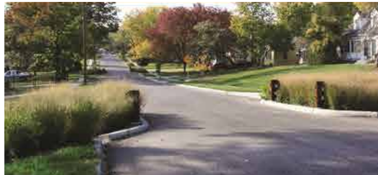
Traffic calming curb extensions and pinch points
