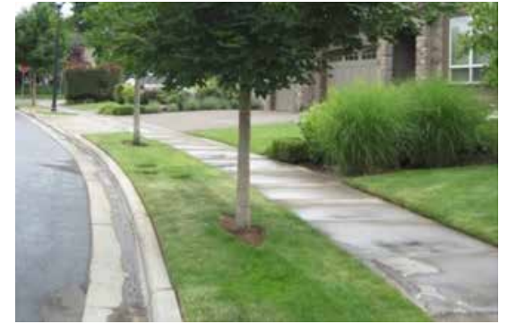
A new sidewalk on the east side of the street
