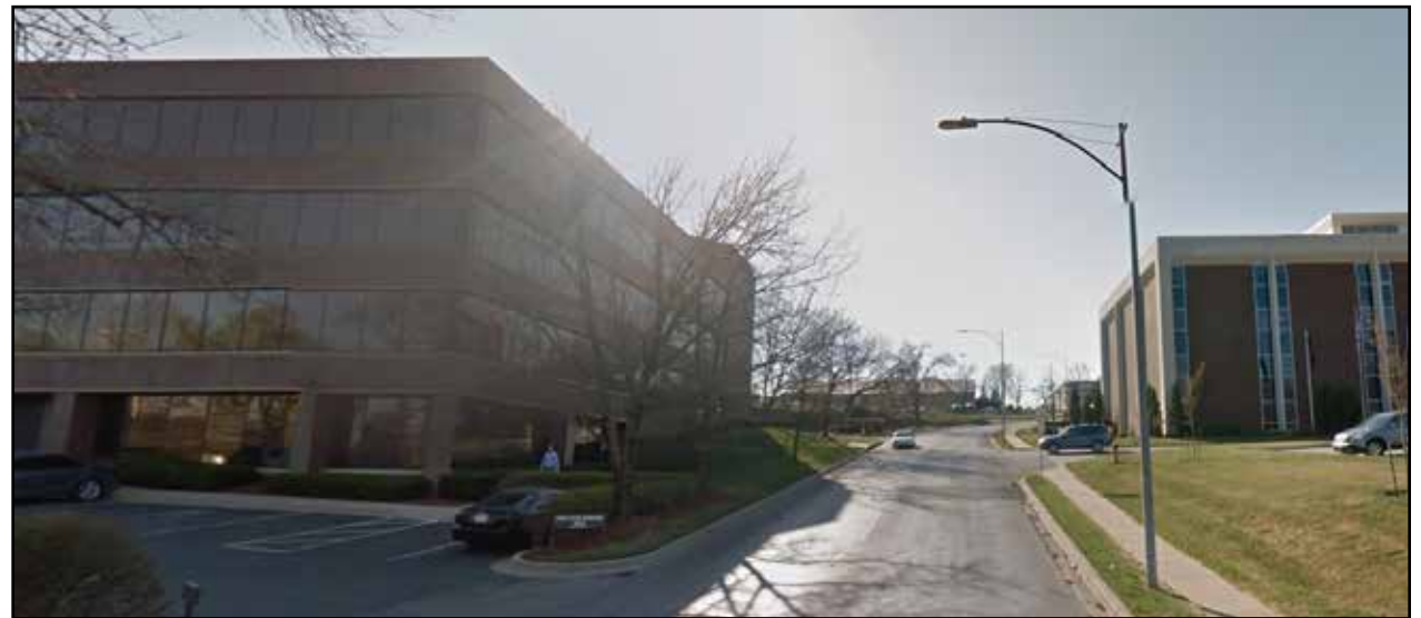
47th Place looking west from State Line Road. The existing street has room to incorporate a new sidewalk on the south side (left).
