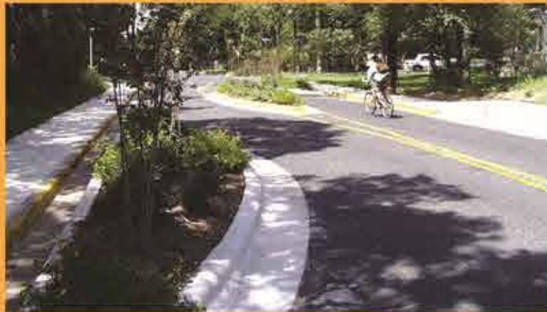
Chicanes (curb extensions)
