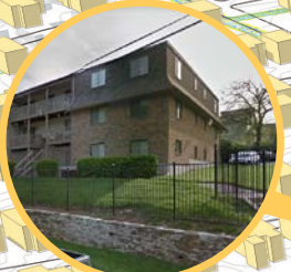
Malvern Hill Apartments
