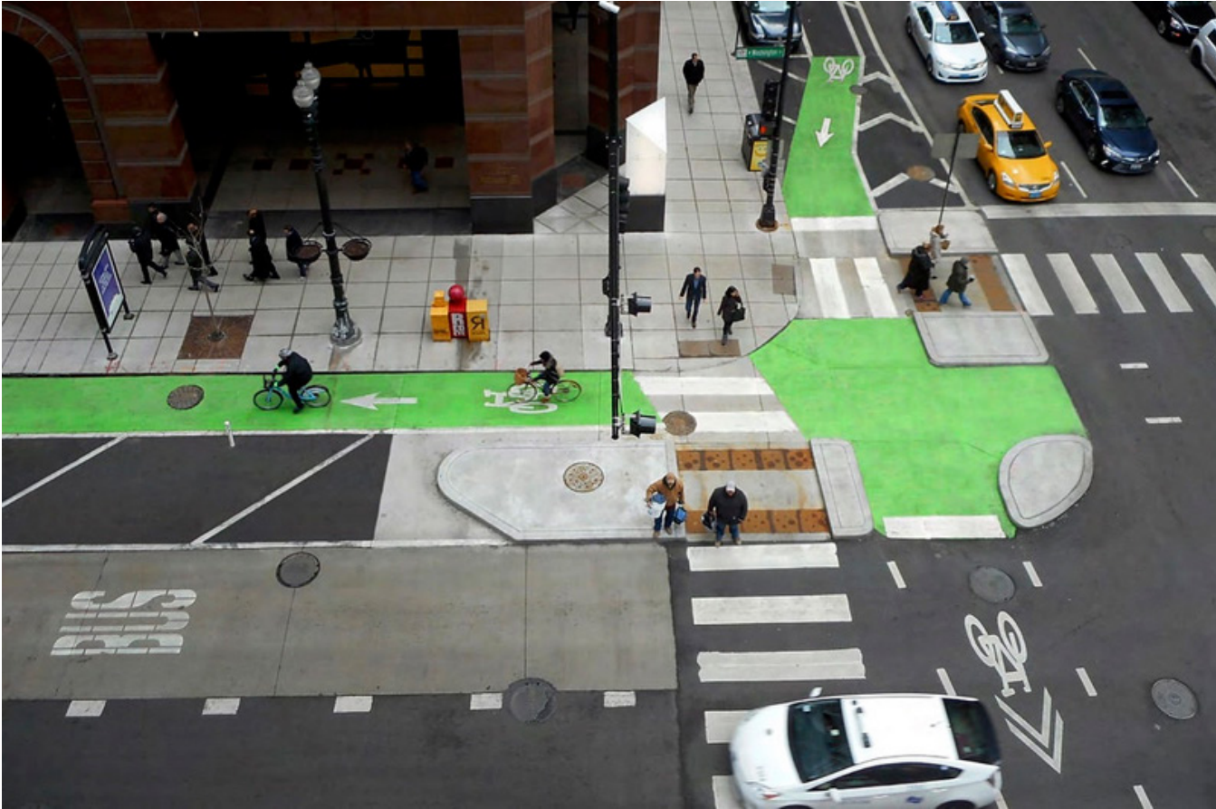
Above: Protected intersection of two one-way bike lanes and a bus-only lane in Chicago. Source: San Francisco Bicycle Coalition.
