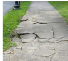
/ Beginning to Deteriorate
